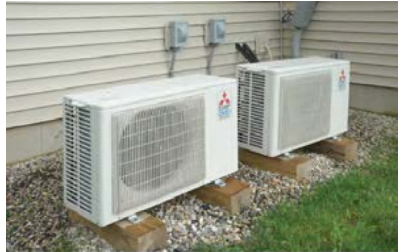
Mitsubishi dual-stage heat pumps produce 92 percent of their capacity at 5°F (minus 15°C) and keep producing heat down to minus 13°F (minus 25°C).
