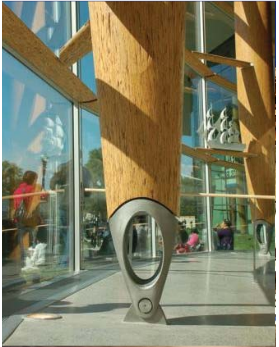
Arena Stage, Washington DC, Bing Thom Architects
