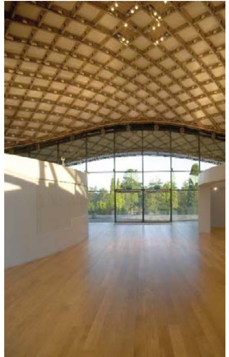
Savill Gardens Gridshell, England Glen Howells Architects
