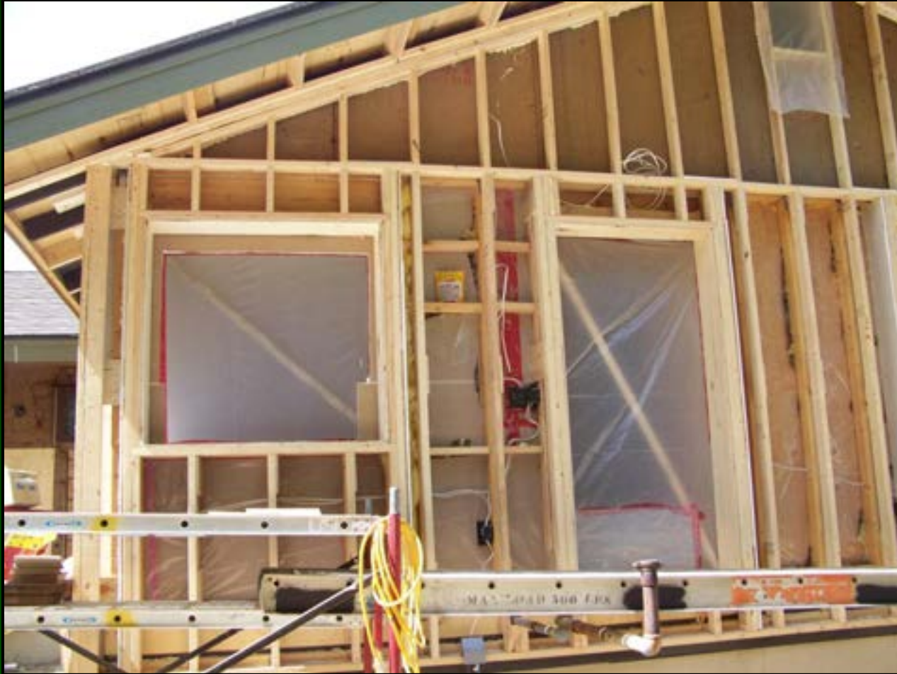
Second wall framed outside of existing wall.
