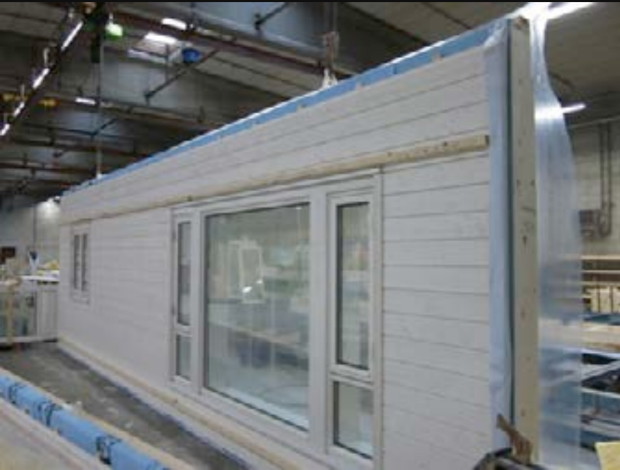
Prefabricated wall panels assembled at Skanska Husfabriken
