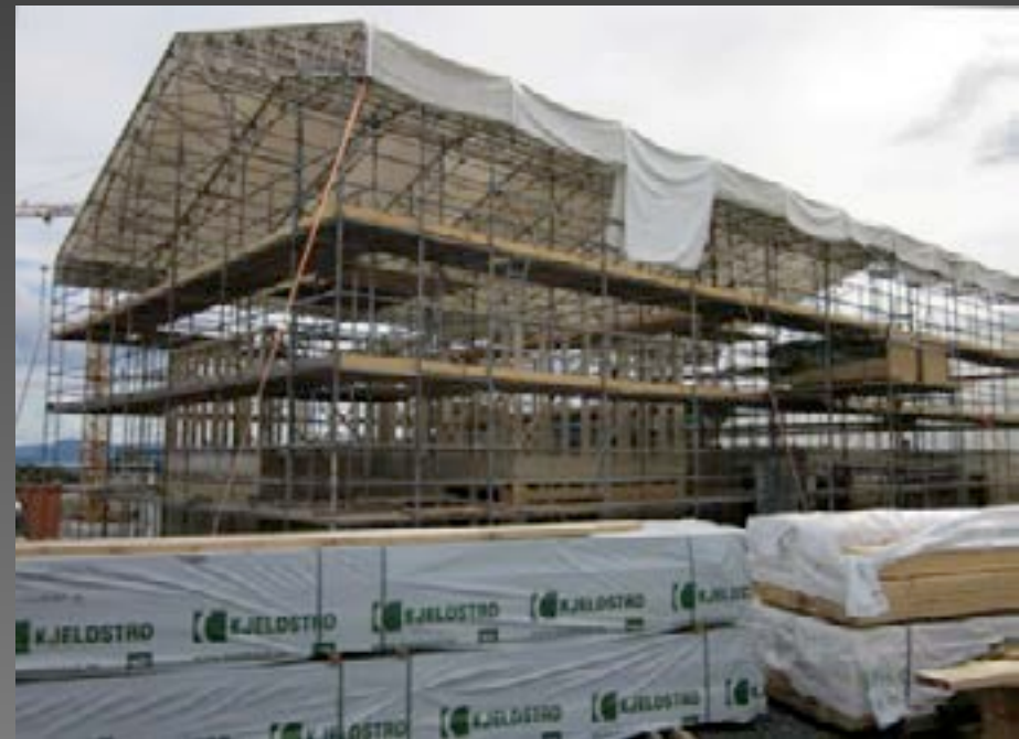
Site construction under temporary shelter scaffolding
