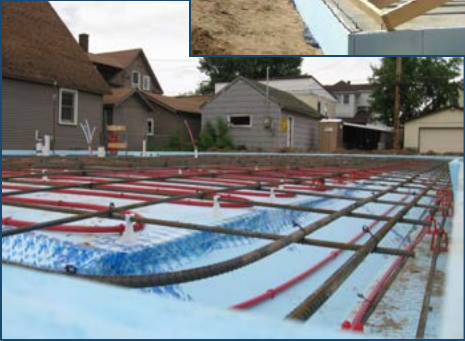
Foundation / slab insulation IECC 2012: R303, R402 ES 3.0: Thermal Enclosure System
