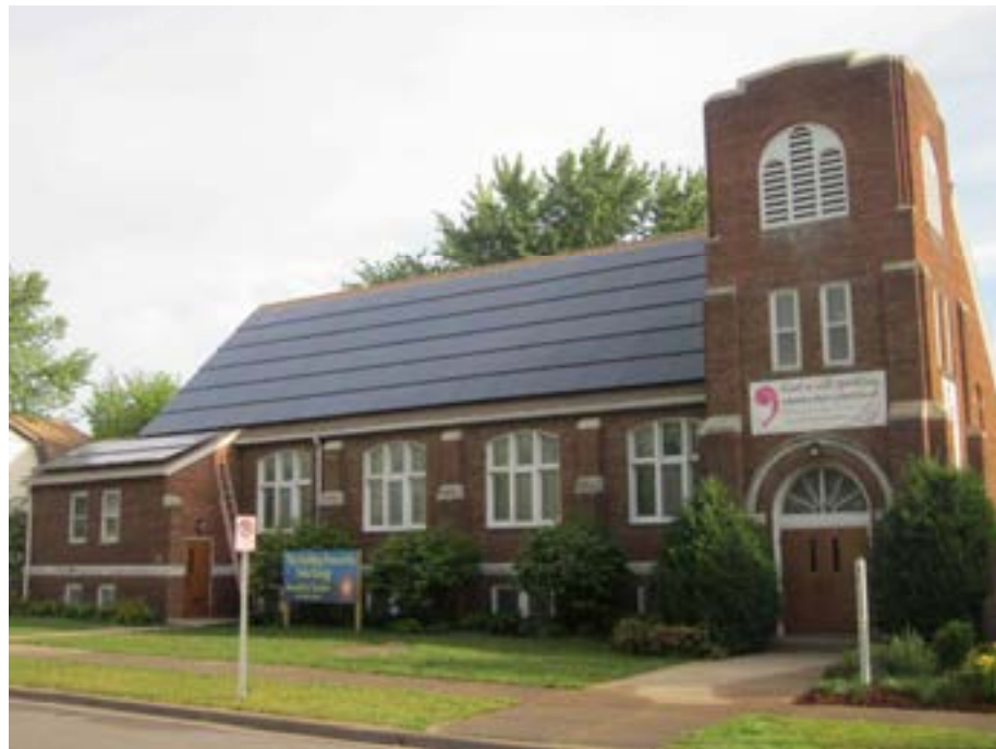
Photo Credit: SunDial Solar; Silicon Energy
