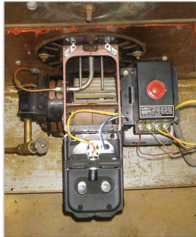
Inspect the Inside
