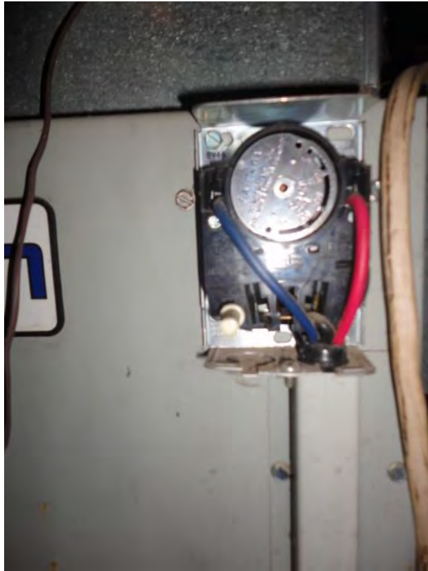
Fan Control with High Limit
