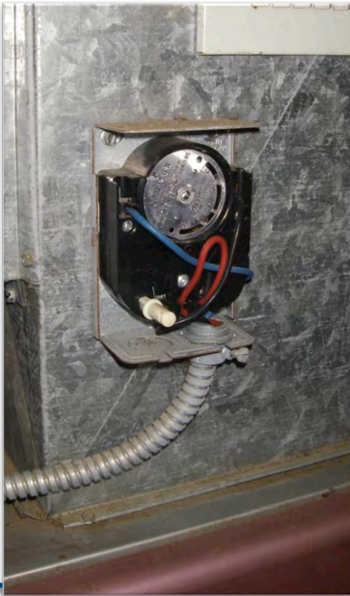
Fan Control with High Limit
