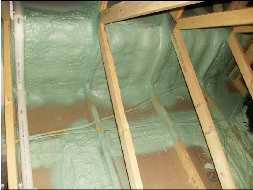
Sealed and insulated short knee wall and top plates
