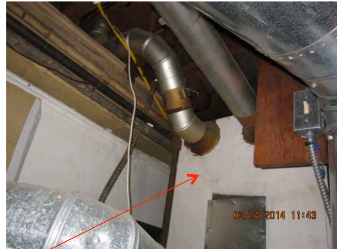
Undersized Ductwork
