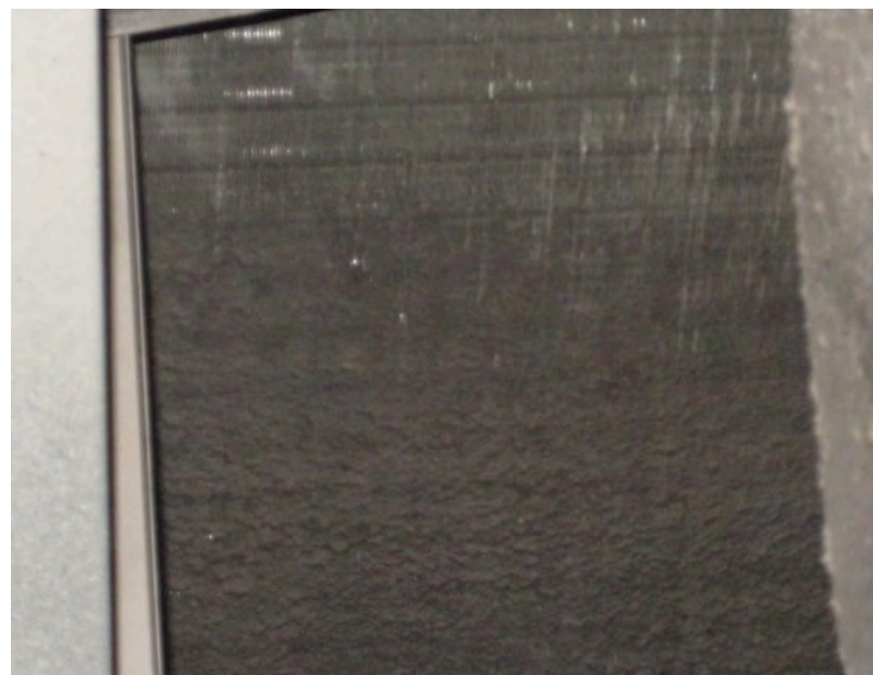
Owner did not know this coil existed
