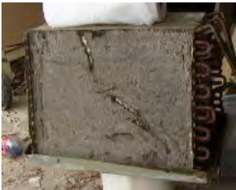
Dirty AC Coils
