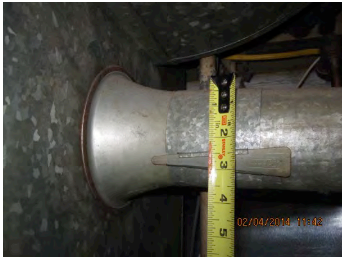
Undersized Supply ducts
