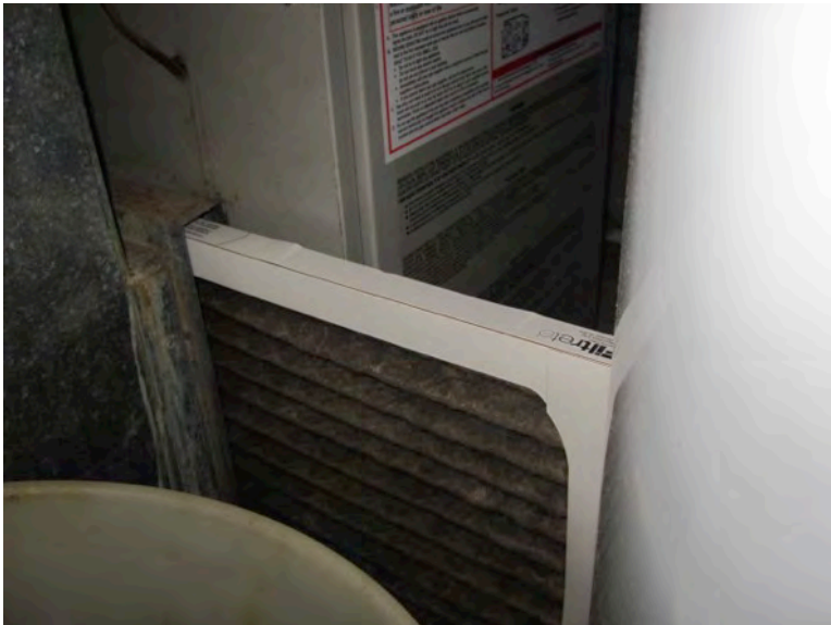
Restrictive filter (up to 50% drop in flow)
