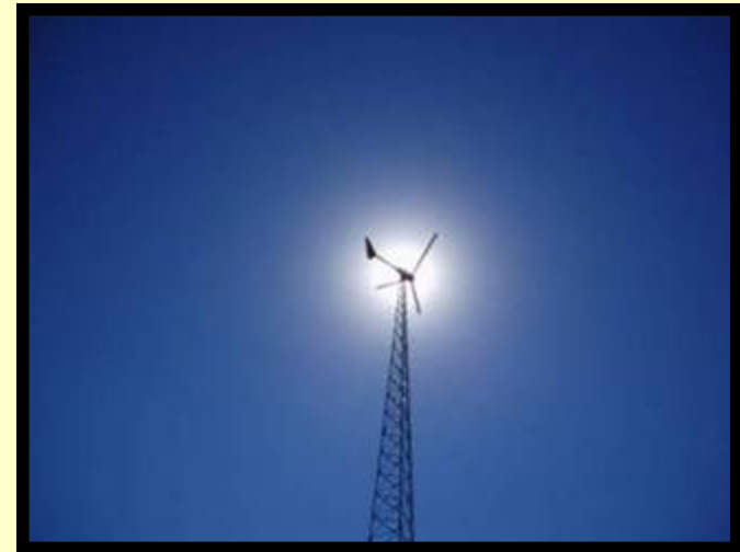
10 kW Grid-intertied Wind Turbine on 120' Freestanding Tower
