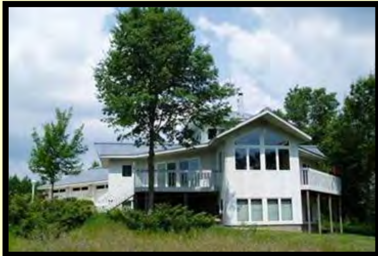
View from South/Southeast
