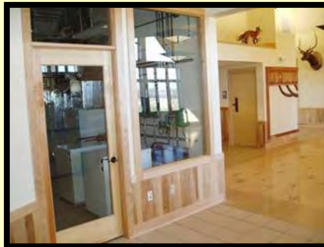
Publicly-viewable Mechanical Room in Lobby
