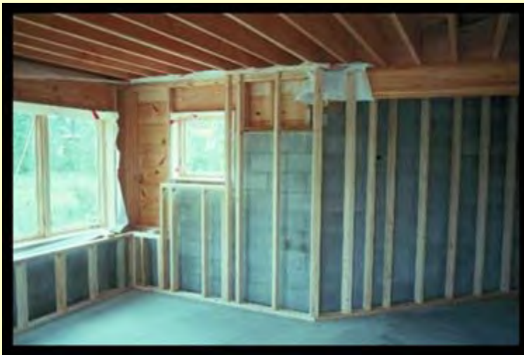
Perimeter Stud Wall @ Foundation Wall & Walkout
