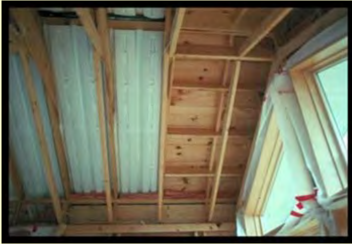
Drop-Rafter & Ventilation Chute
