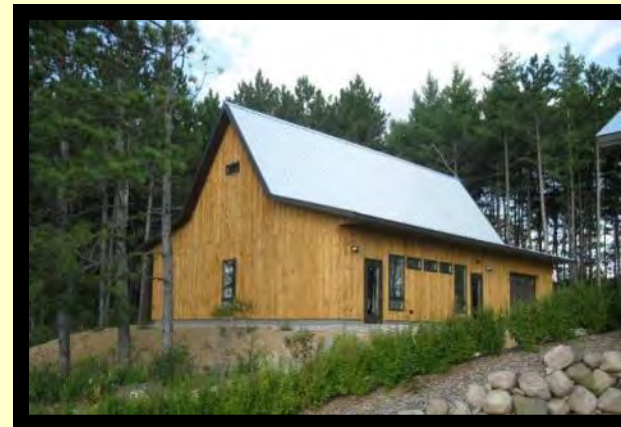
MREA Renew the Earth Institute North training Building
