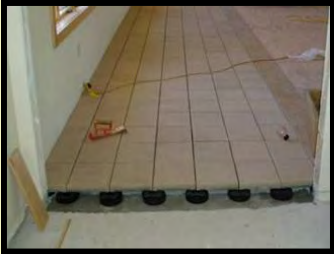
Depressed Floor Slab with Raised “walk-off” Paver Tiles
