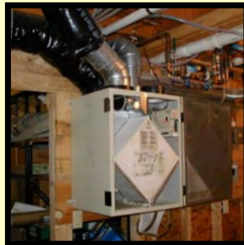
Heat-recovery Ventilation Unit
