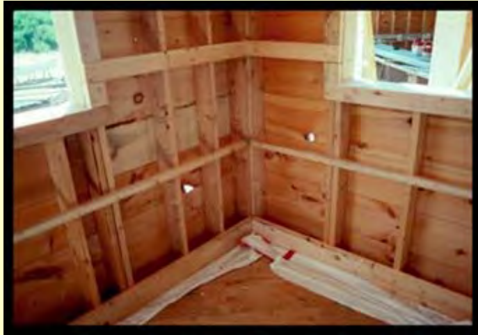
Interior Horizontal Strapping
