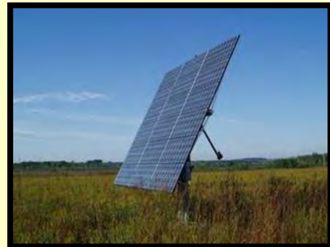
2.3 kW Tracking Array Solar Photovoltaic Grid-intertied System
