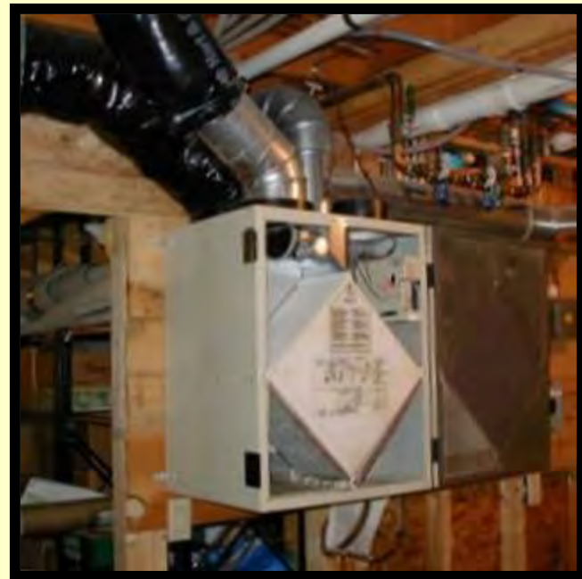
Heat-recovery Ventilation Unit
