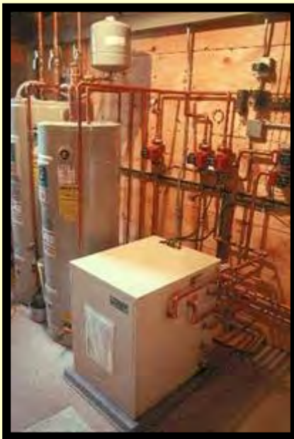
Ground-Source Heat Pump Unit
