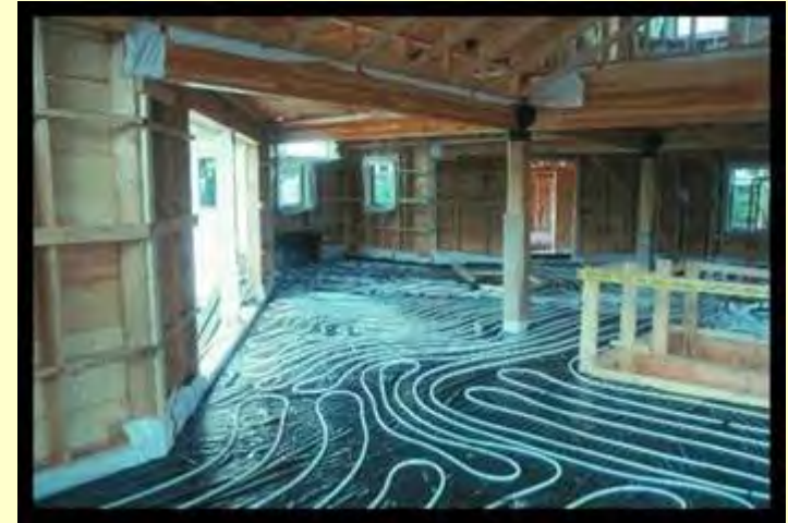
Hydronic-Radiant Tubing Layout @ Living
