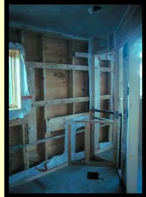
V.B. Detail @ Partition/ Exterior Wall Strapping
