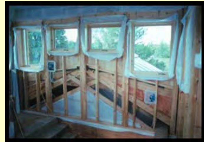
Loft/ Drop-Rafter/ Window V.B. Detail
