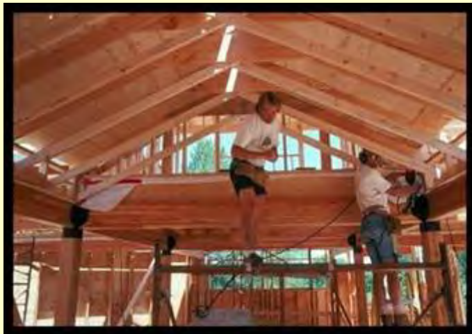
Sloped Ceiling/ Drop-Rafter
