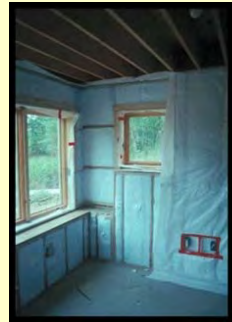
Insulated Perimeter Stud Wall @ Foundation Wall & Walkout
