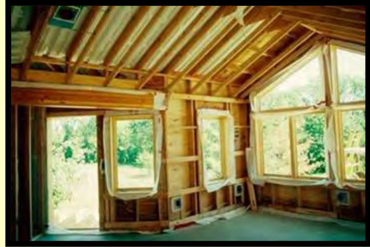
Interior Strapping & Drop rafters
