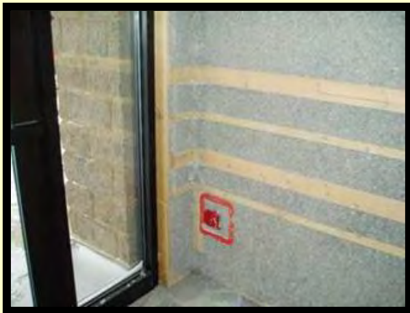
Electrical Box/ Airtight Enclosure/ Interior Strapping/ Spray-cellulose Insulation
