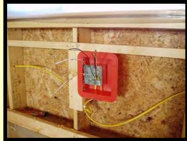
Airtight Electrical Box Enclosure
