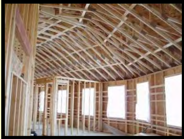
Interior Strapped Wall w/ Raised-heel Roof Truss
