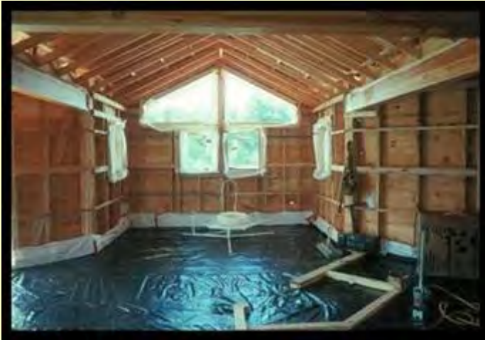
Main Floor Hydronic- Radiant Slab Prep
