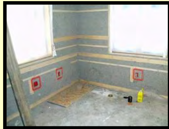
Electrical Box/ Airtight Enclosure/ Interior Strapping/ Spray-cellulose Insulation
