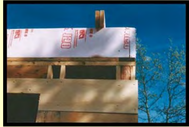
2" Rigid Insulation @ Upper Rim Joist
