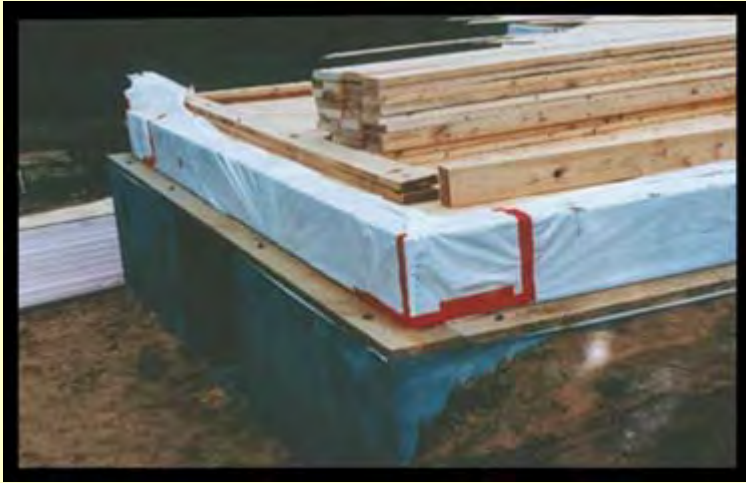
Recessed Rim Joist @ Main Level
