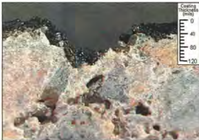
Asphalt emulsion at 40 mil dry thickness on concrete block
