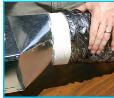
Mechanically fastened and sealed.
