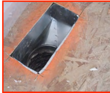
Boot to floor connection not sealed.
