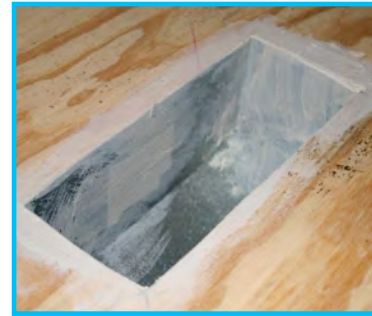
Boot to floor connection sealed.
