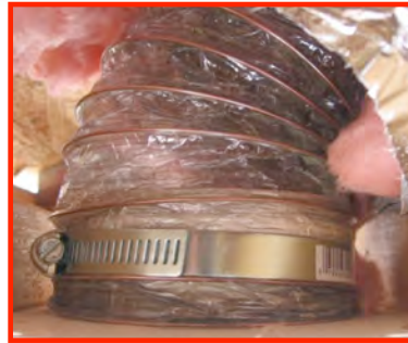
Connection in place but not sealed.
