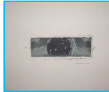
Boot to drywall connection sealed.
