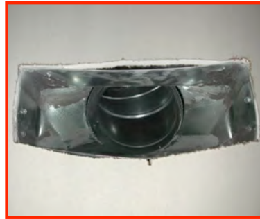
Boot to drywall connection not sealed.
