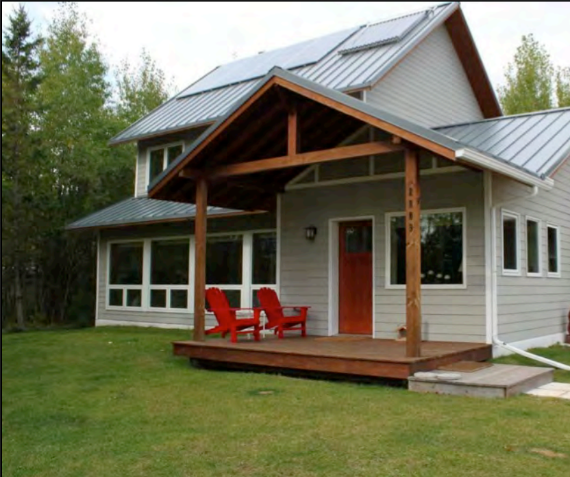
Integral roof overhangs For taller windows (lower sill), overhang may need to be deeper
