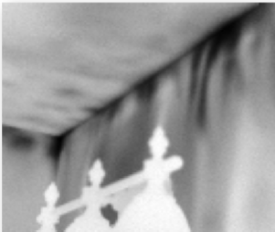
Attic air infiltration into the wall
