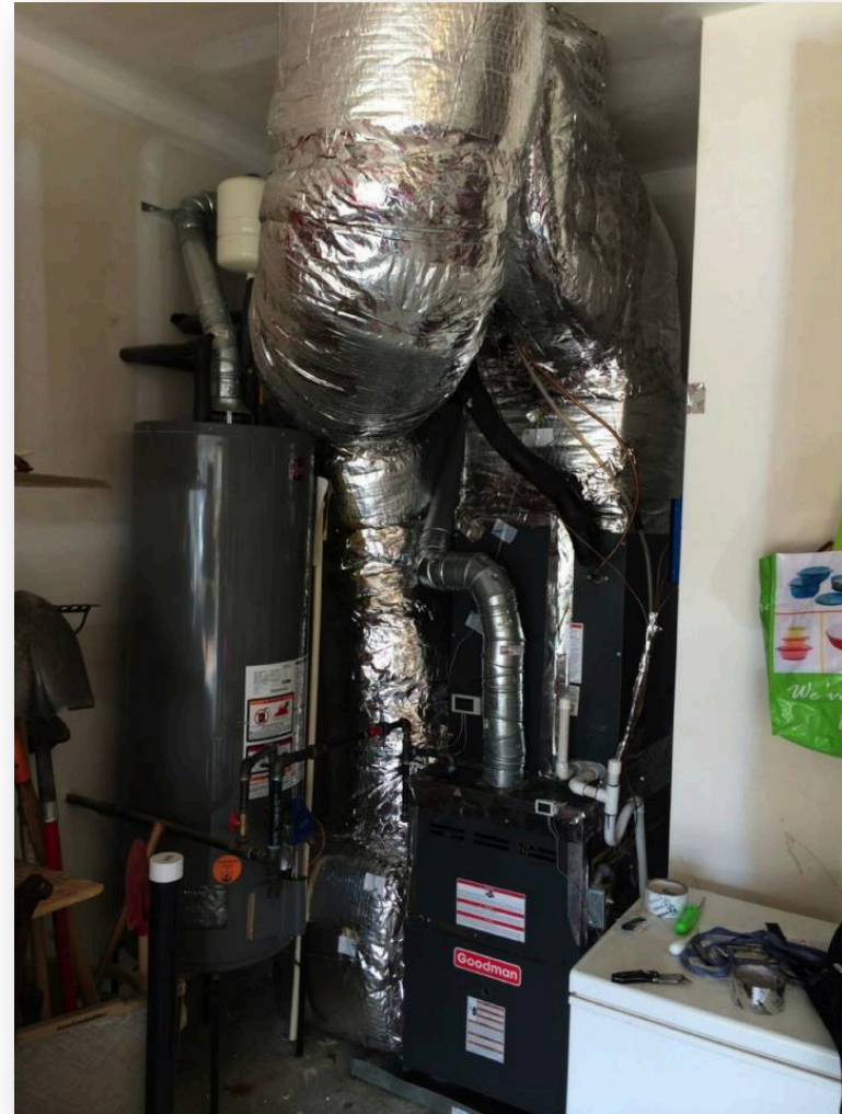
Picture Source: Construction Instruction
