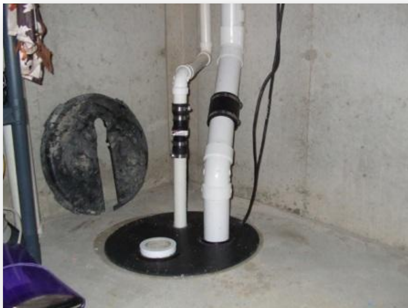
Sealed Sump Pump
