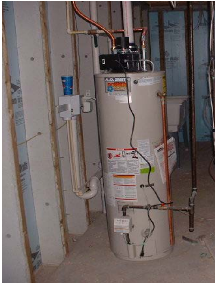
Power Vented Water Heater
