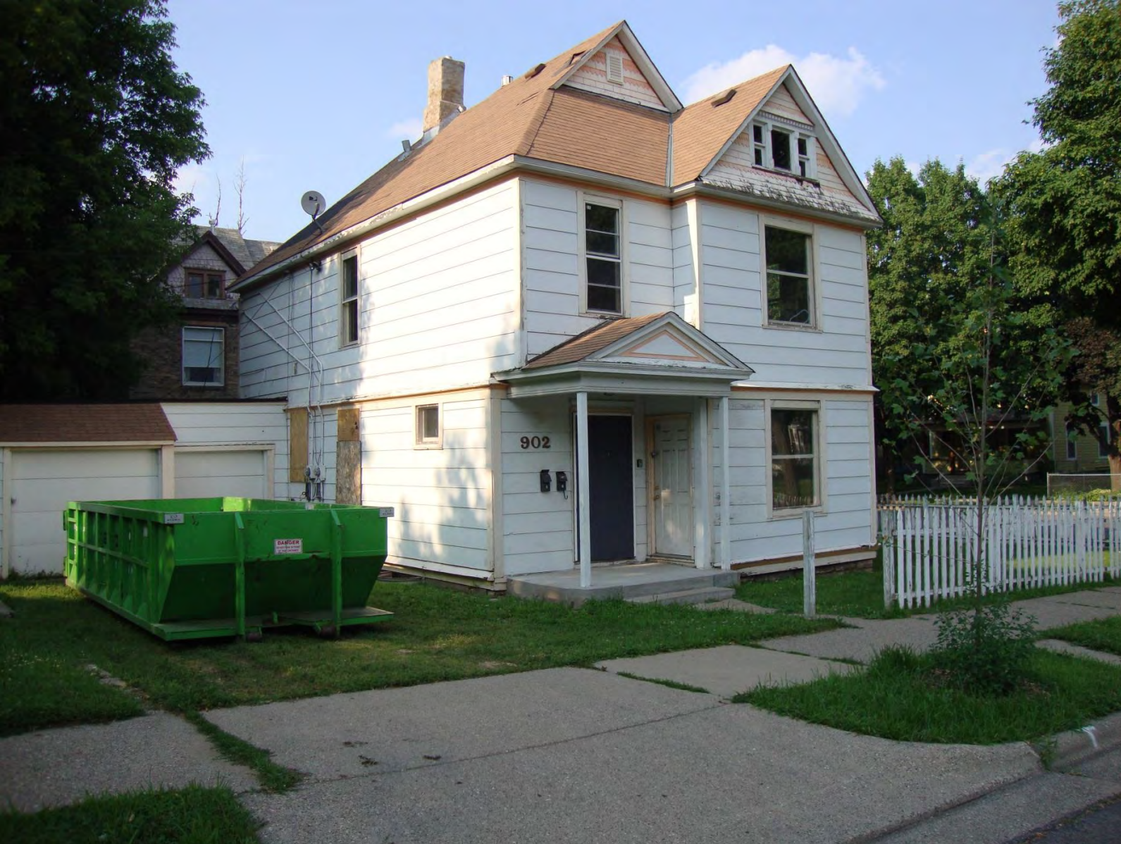
Rehab test house owned by Urban Homeworks
