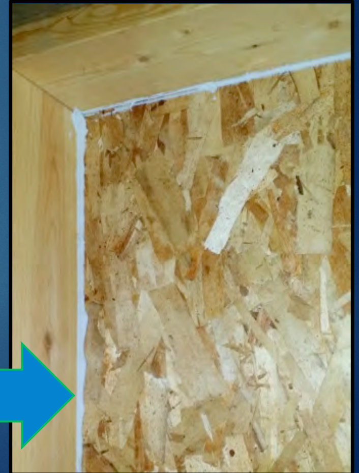
Caulking the framing
