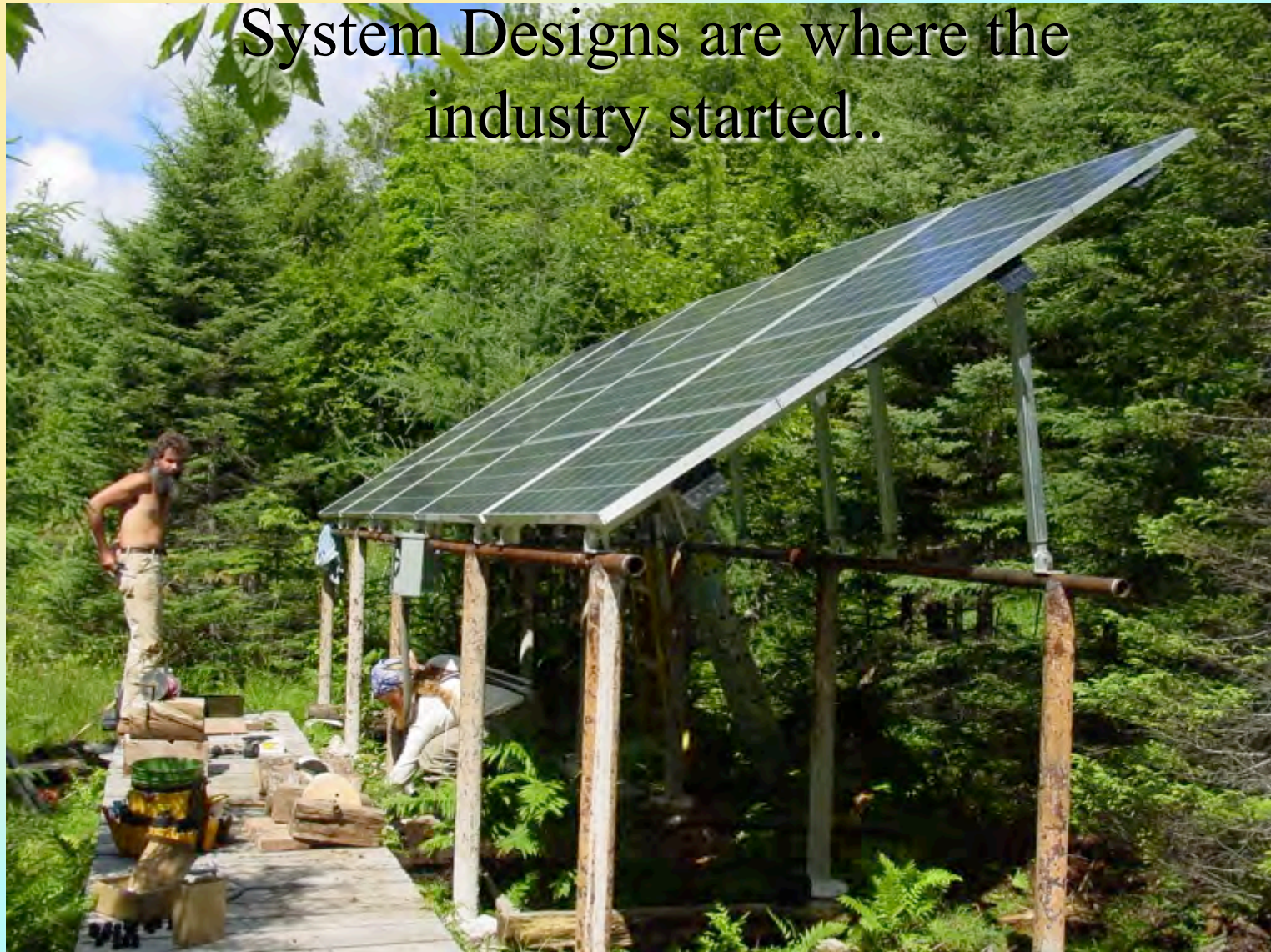
SunDance Homestead, Upper Peninsula Michigan Off-Grid Battery Based Stand Alone System 2400 watt PV Array, 5.5Kw Inverter, 1050Ahr Battery
