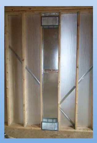
Avoid Ductwork outside conditioned space
