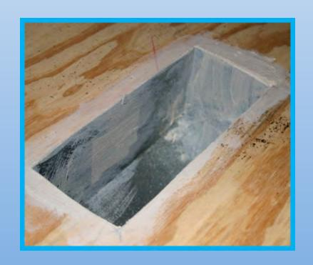
Total Duct leakage testing will be required to be 4 CFM per 100 sq.' of conditioned floor area.
