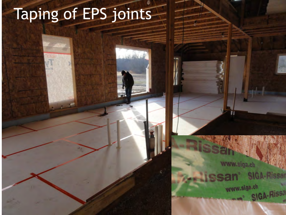
All penetrations sealed with SIGA tape.
