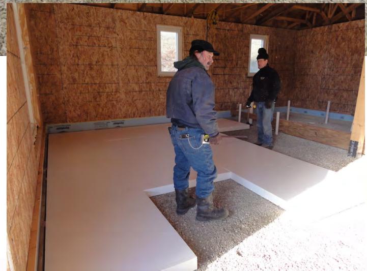
Installation of high density EPS insulation - 3 perpendicular layers
