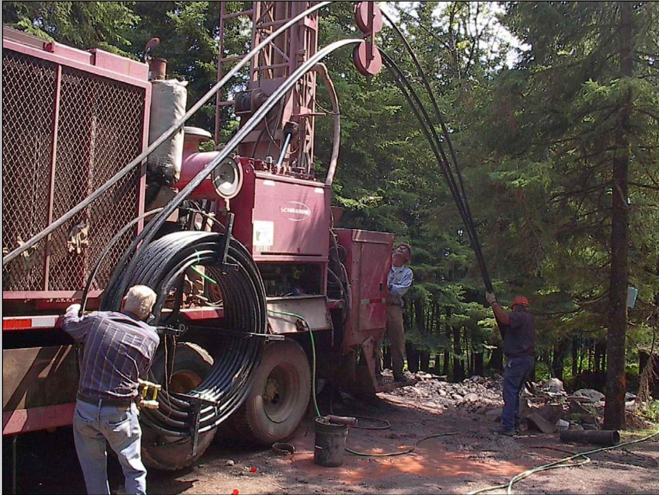
Vertically Bored in Rock
