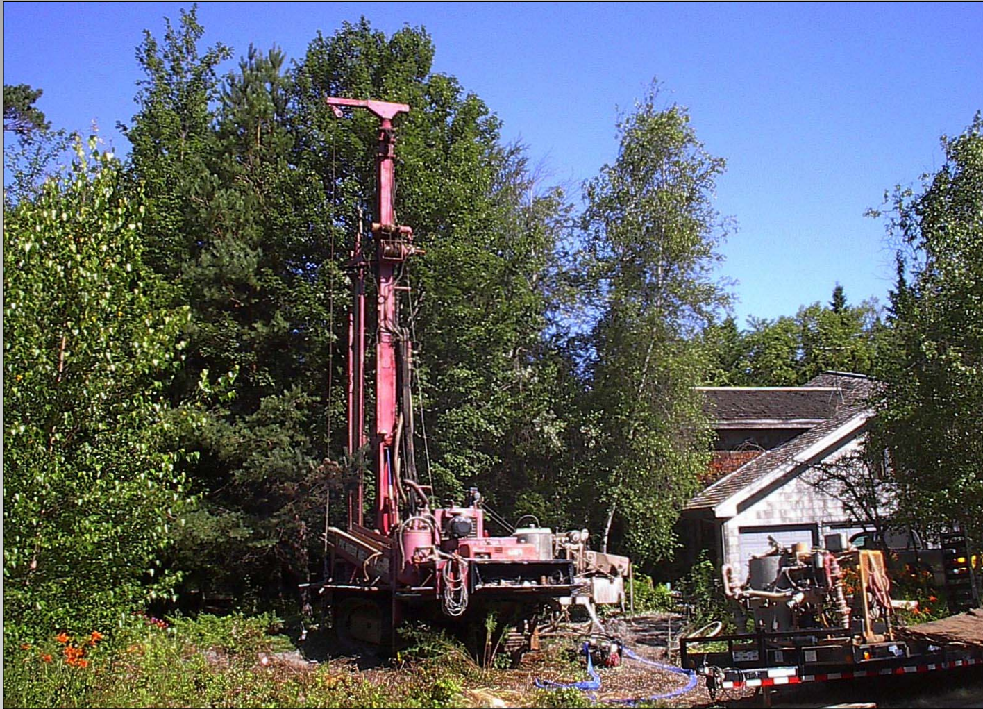
4.0<7T Vertically Bored GHP System @ 62.2% GHP Sizing
