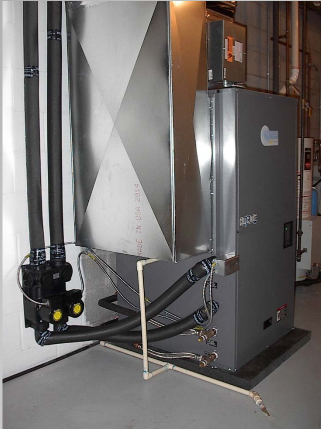
State-of-the-Art 2-Stage Forced Air GHP System Installation
