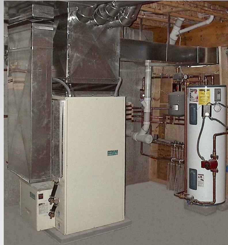
Older Generation Stand-Alone Combined F/A & HYD GHP System
