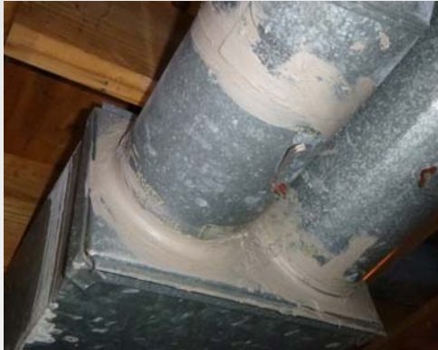
Applying mastic and foil tape to duct work
