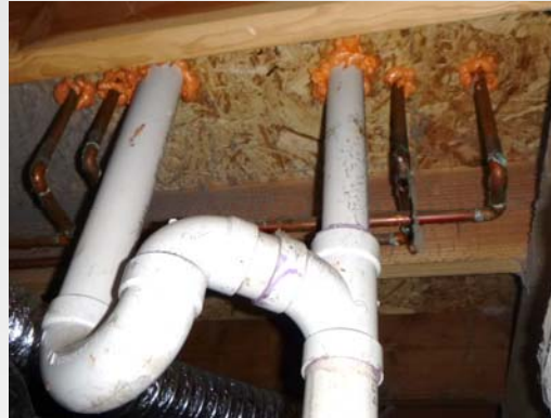
Expanding urethane foam at penetrations beneath the floor
