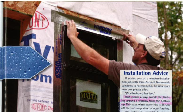
Proper installation of flashing around a window opening is crucial to prevent water infiltration.
